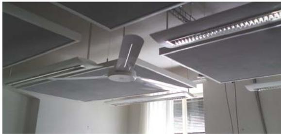
Figure 3 Ceiling fan and suspended ceiling with PCM in R3
